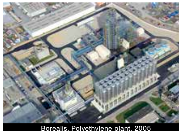
Borealis, Polyethylene plant, 2005
