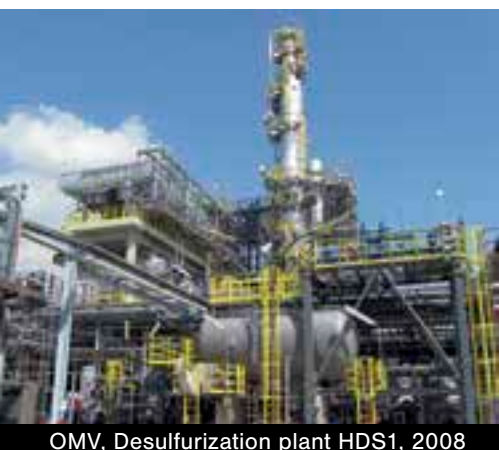
OMV, Desulfurization plant HDS1, 2008
