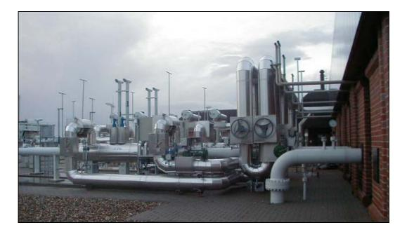
Fig. 3 - Station piping UGS Nuettermoor
