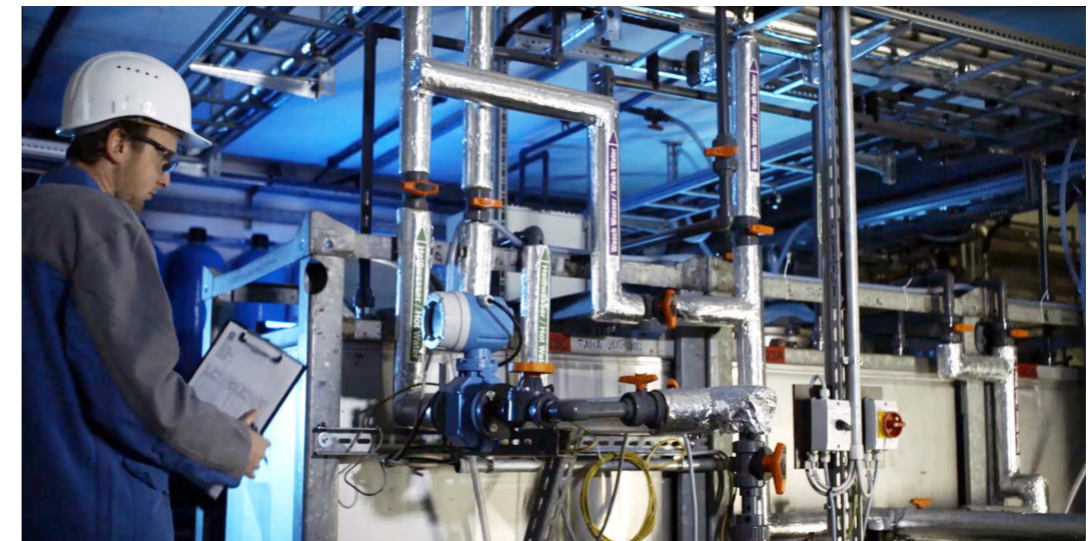
Our Pörner experts support you from feasibility to full-scale plant implementation.
