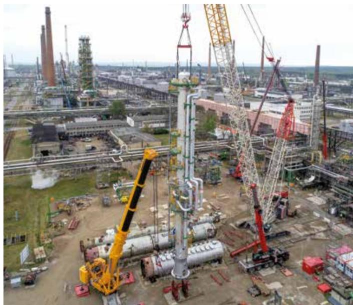
**Aromatics extraction plant at the PCK refinery: Classic revamp with minimization of energy and operating material consumption combined with innovative EDL technology for extractive distillation to minimize of toxic solvents.**
