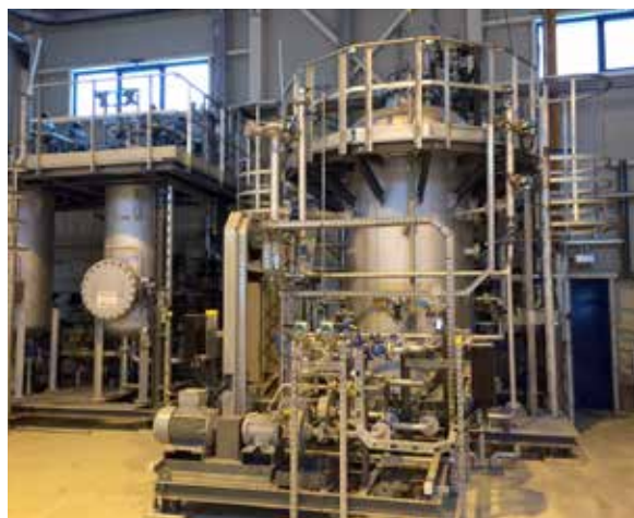
Supply of a produced water treatment plant with subsequent re-injection into the reservoir with a capacity of 41.6 m 3 /h (Tazlău / Romania, executed on behalf of Siemens)
