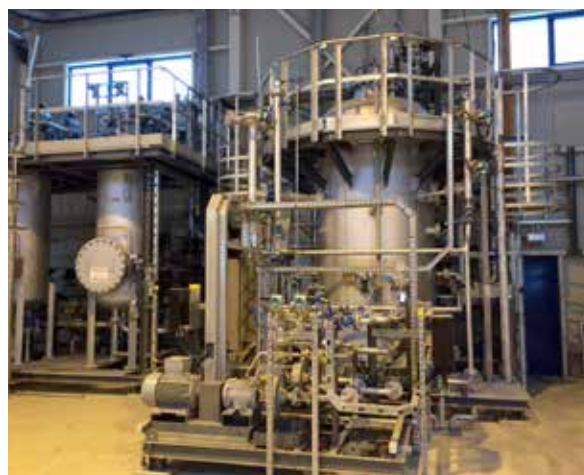
Supply and commissioning of a combined produced water treatment plant with a capacity of 41.6 m 3 /h and surface water treatment plant with a capacity of 33 m 3 /h with subsequent re-injection into the reservoir (Tazlau / Romania, executed on behalf of Siemens)
