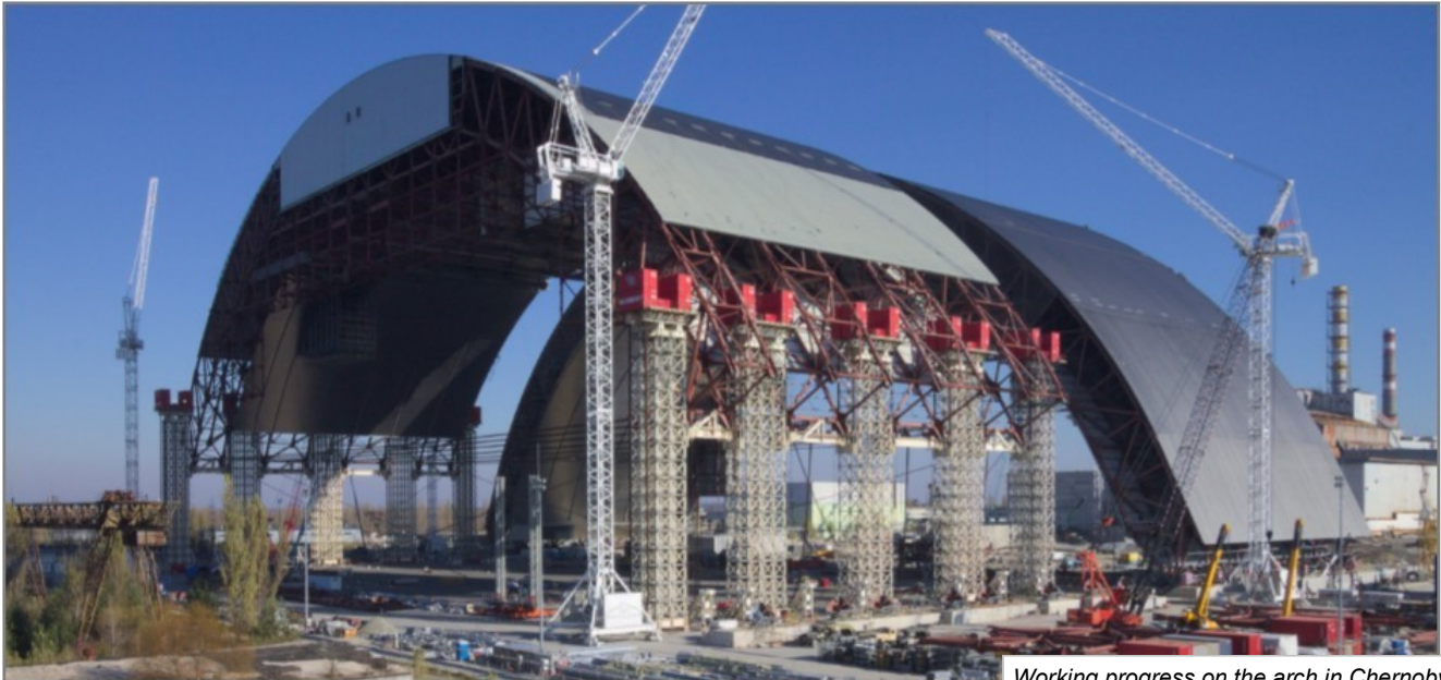
Working progress on the arch in Chernobyl
